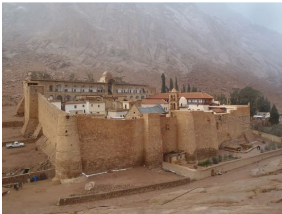
Figure 3: The walls of Saint Catherine's.
